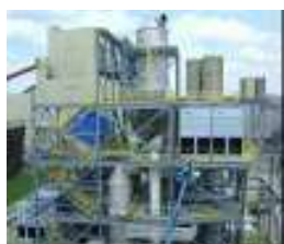
AEP Mountaineer US - 58 MWth Chilled Ammonia, coal
