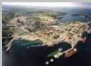
TCM Mongstad Norway - 40 MWth Chilled Ammonia - Gas
