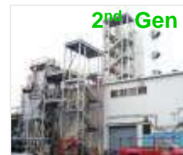
DOE/Alstom Windsor US - 3 MWth Chemical looping - coal
