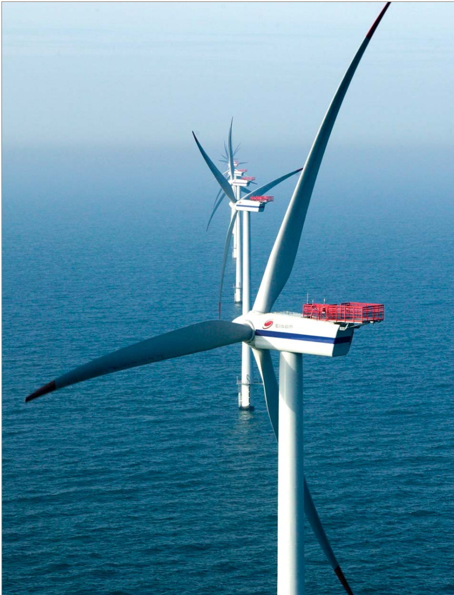
Fig. 10. The Vestas V80 2 MW turbines at Horns Rev need 4 m/s wind speed before they can begin generating but must feather their blades at around 25 m/s to prevent mechanical damage (copyright: Elsam A/S)
